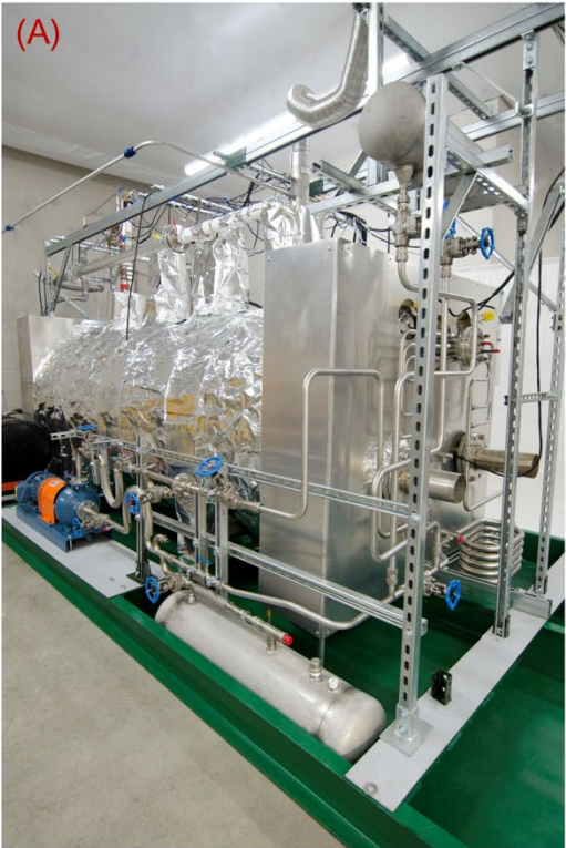
Snapshots of sulfur-TES technology: (A) 350-kWh sulfur thermal-energy storage (TES) prototype at Element 16 facility; (B) Engineering drawing of sulfur TES illustrating charge (red pipe) and discharge (yellow pipes) heat-exchanger circuit within molten sulfur; and (C) 3D computational simulations of the time variation of temperature contours at a cross-section of sulfur TES during charge process.
